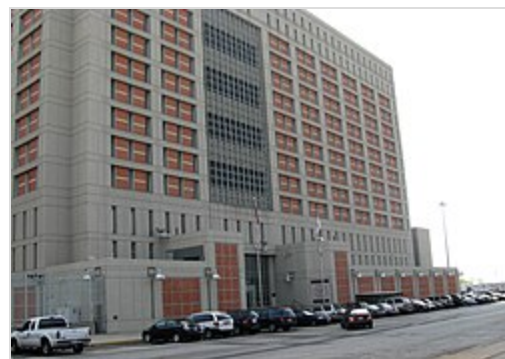
The Metropolitan Detention Center , Brooklyn , in New York City
